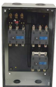
Interior View of ML SASD
