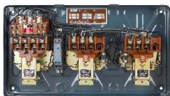
Interior View of MK2 FASD
