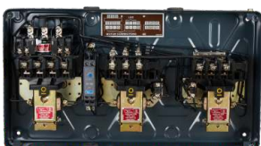
Interior View of MK1 FASD
